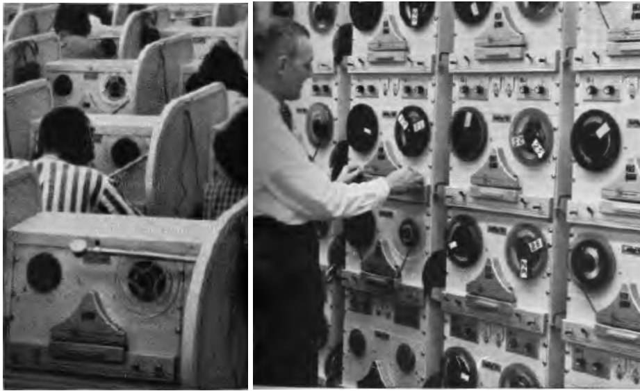
Figures 2.7 and 2.8. Both types of listening laboratories located at Duke University. (Left). Tape recorder is located in each study carrel. (Right). Tape recorders are centrally located and broadcast to study carrels. Source: AudioVisual Instruction. Dept. of Audiovisual Instruction, National Educational Association. Washington D.C. Dec 1964. Pp. x.
